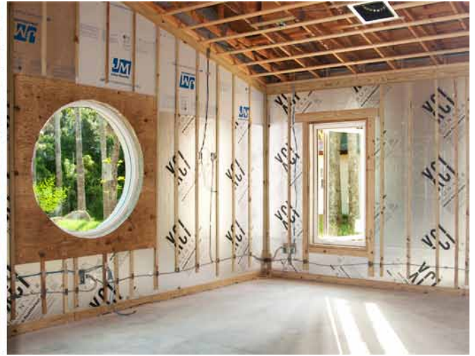
PIAS office under construction.
