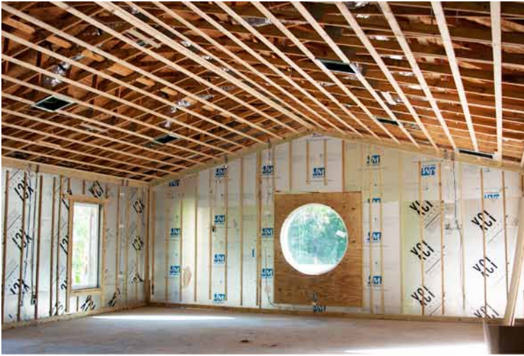
Audubon House Classroom under construction.
