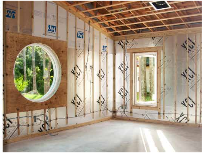
PIAS office under construction.
